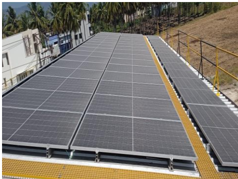
Tilted- Roof top Solar Plant
